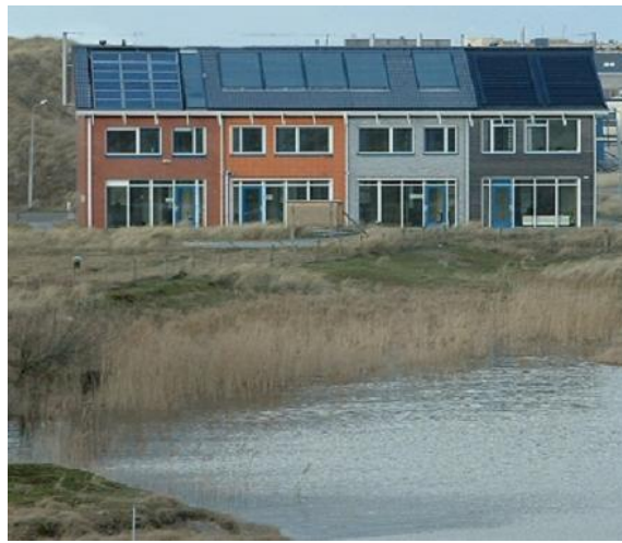
Figure 5: The four single family dwellings. The second house to the left is used for measurements with the adsorption chiller
